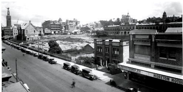
ANZAC square under construction circa late 1920's
