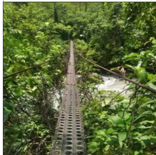
Marsden Matting on a footbridge over the Guama River, Kabwum, Morobe Province PNG.
