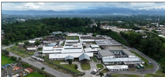
The new Australian Government funded ANGAU Memorial Hospital, Lae.
